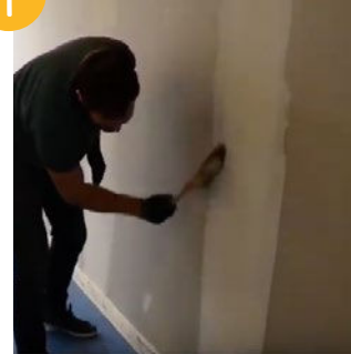
CLEAN THE AREA BEFORE THE INSTALLATION
